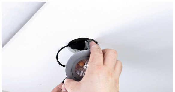
5 - inserting the spotlight into the ceiling cut-out
