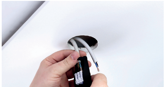
1 - fast wiring / through-wiring on the quick connection box thanks to screwless plug-in terminals
