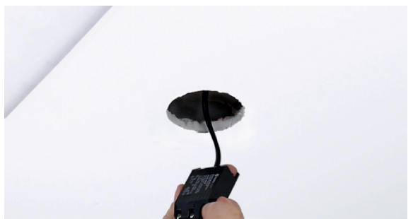
3 - compact power supply unit is inserted into the cavity
