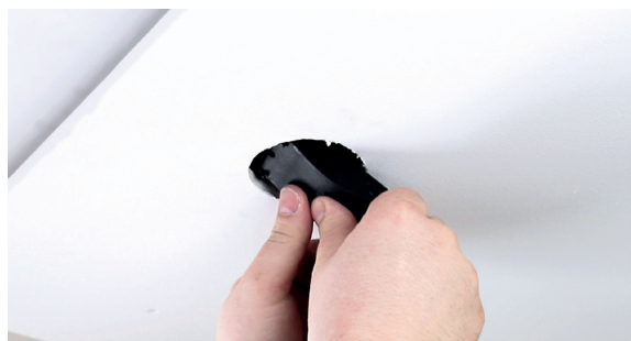
2 - quick connection box is placed through the 68 mm cut-out in the cavity
